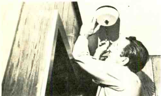
HEAT AND SMOKE DETECTOR added to Westinghouse system protects against fire in addition to basic intruder protection.
